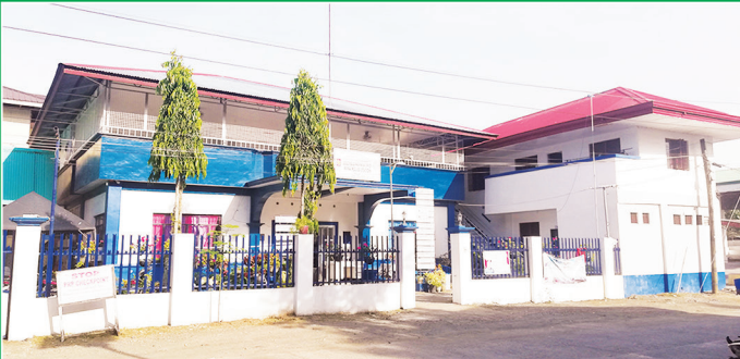
Mina Municipal Police Station
