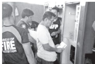
15 November 2016. An ocular inspection of the newly issued SINO-JIANGTE Fire Truck and its Auxiliary Equipment, Tools and Accessories conducted by F/INSP MARIO L LAÑA, BFP, together with FO3 Alberto G Salita Jr, FO3 Jemboy B Pacardo, FO2 Marugerald Sapitanan and Mr. Julian G Gutierrez, COA Senior Technical Audit Specialist of COA Central Office, at Mina Fire Station.
