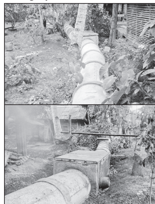
Construction of R.C. Pipe Drainage System
