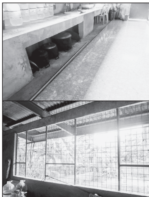
Repair of H.E. Kitchen of Mina Central Schools
