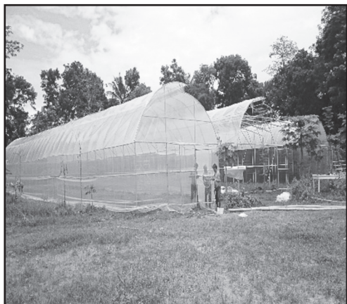
Construction of 2 units greenhouse
