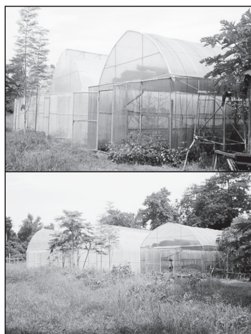
Construction of GREEN HOUSE SYSTEM
